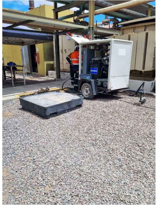
Transformer Maintenance Oil Filtration and De- gasification North QLD 2022
