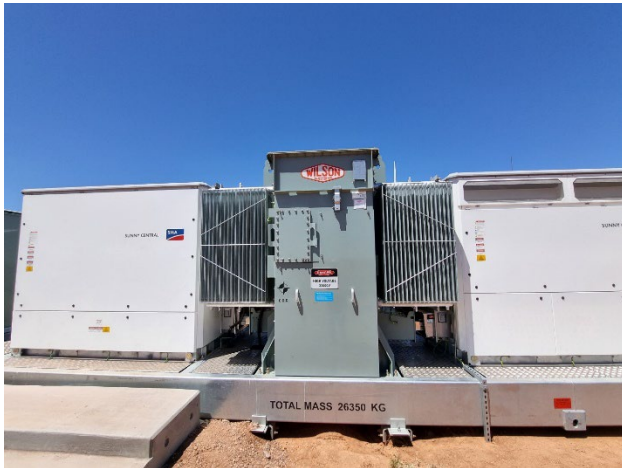
PCU HV Testing and Commissioning SA ESB Power 2022
