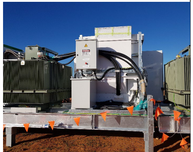
Final Installation of PCU after delivery
