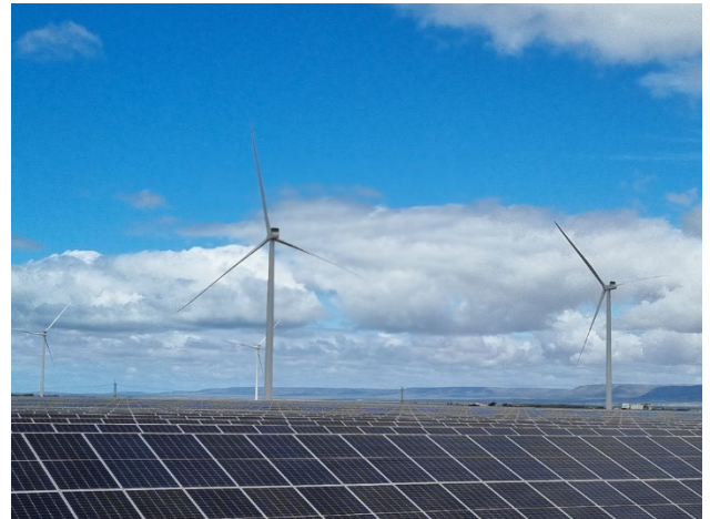
Renewable Hybrid Plant Solar and Wind Farm SA HV testing ESB 2022
